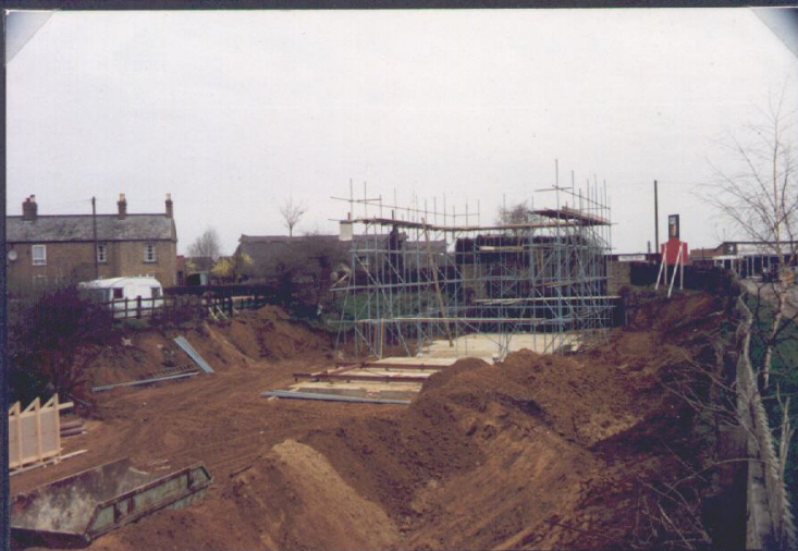
Construction by 'POTTON'
