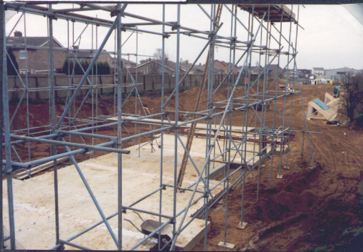
Many tons of sand were brought onto the site .
