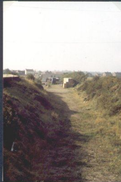
Former railway track, looking South
