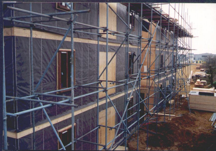
The rooms were placed in position as complete units.
