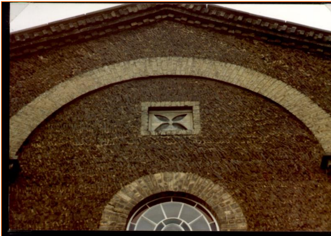
Herringbone ironstone facing on the former Congregational Chapel
