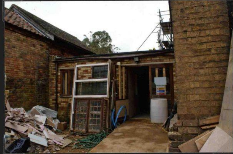
ENTRANCE TO FLATS
